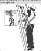
Attach rope tethers around pole or to structure. Apply tension..
