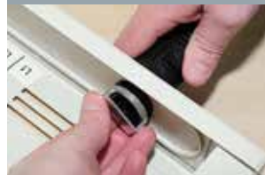
FLP conduit with sheath trimmed back
