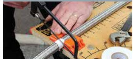
Cutting of overbraided conduit is made much easier by tightly wrapping self adhesive tape around the conduit and sawing through the middle of the tape. The tape should be removed if EMC screening is required. Ensure you make a straight vertical cut.
