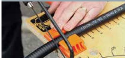
Metallic conduits should be cut with a fine tooth (32 TPI) hacksaw or bandsaw. Ensure you make a straight vertical cut. Our clamping vice, part no. BSB makes the use of a hacksaw much easier.
