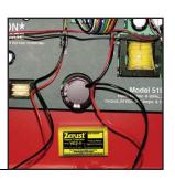
A ZERUST® VC6-1 VAPOR CAPSULE PROTECTING AN ENTIRE CONTROL ROOM FROM CORROSION.
